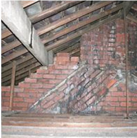
Incomplete party wall (left) and complete (right)
